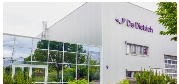
De Dietrich Besigheim, Germany
