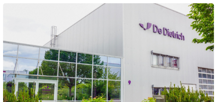
De Dietrich Besigheim, Germany
